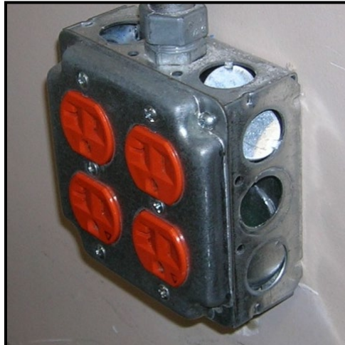
Figure 1-6.--Missing Knockouts
