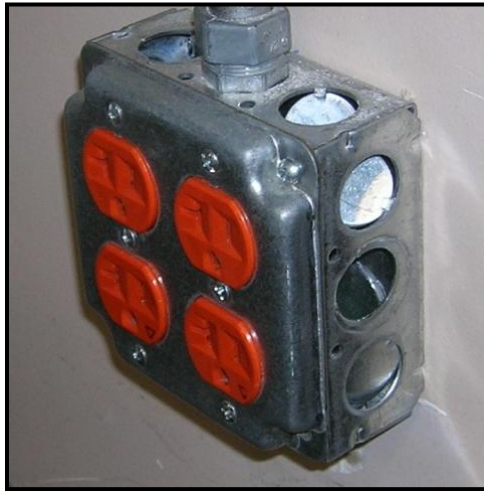
Figure 1-6.--Missing Knockouts
